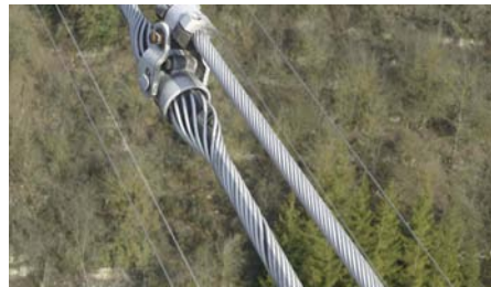
Inspection of power lines
