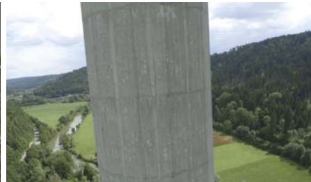
Inspection of bridges
